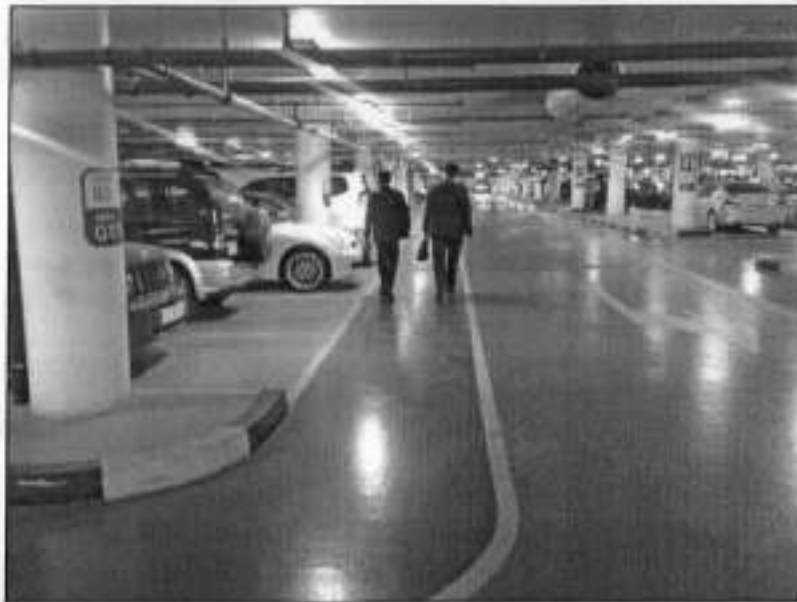
Figure 3.21: Driveway with Pedestrian Strip
